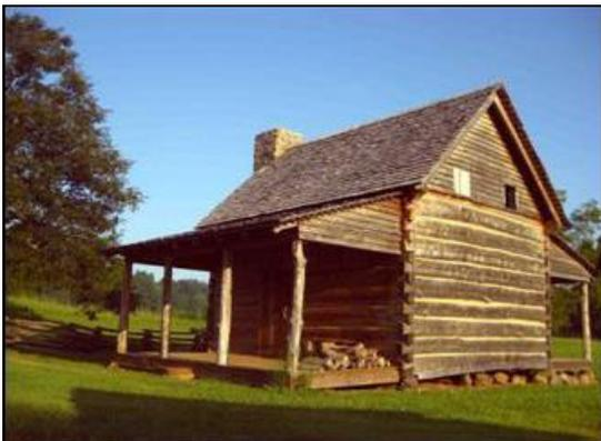
Gaps between logs are filled with "chink". 'Perma-chink' is a commercial brand. The classic formula for making chink is: 3 parts dirt, 3 parts sand and 2 parts Portland cement with an appropriate amount of water. It is best to let the stacked logs sit for a year before chinking them.
